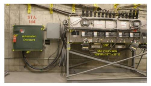
Figure 25—Submersible S&C Vista 5-Way Switchgear and Automation Controller
