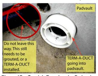
Figure 67—Conduit Entering the Padvault
