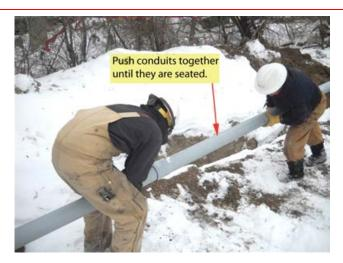
Figure 26—Seating the Conduit
