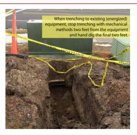
Figure 5—Trench to Energized Equipment
