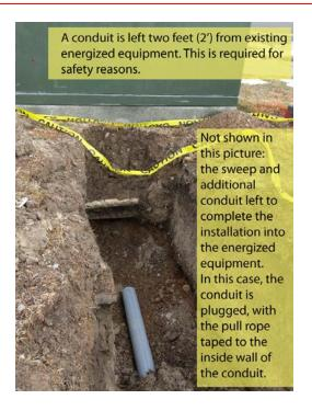
Figure 23—Installing Conduit to Existing (Energized) Equipment
