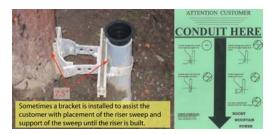
Figure 3 I—Riser 7.5" from Pole, Bracket and Power Company Template
