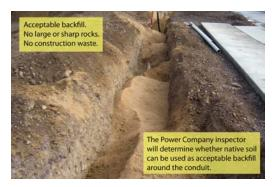
Figure I5—Acceptable Backfill
