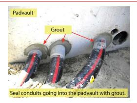
Figure 69—Grout Used for Conduit Entering the Padvault
