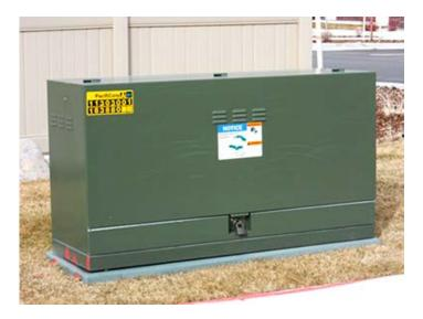
Figure 48—Three-Phase Sectionalizing Cabinet
