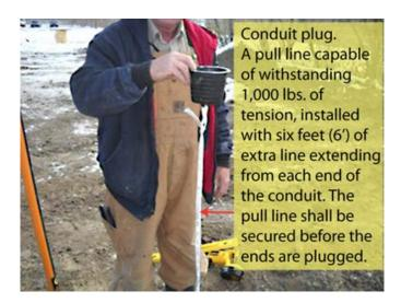
Figure 27—Conduit Plug and Pull Line
