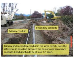
Figure 9—Primary and Secondary Conduits in Trench
