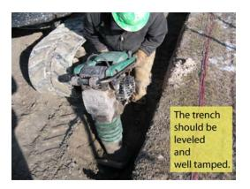
Figure 14—Typical Conductor Trench
