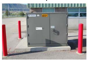
Figure 40-Barrier Posts, Example
