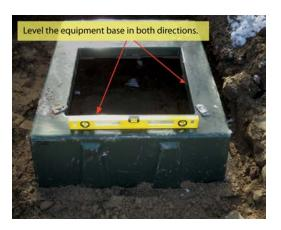
Figure 37-Leveling the Equipment Base
