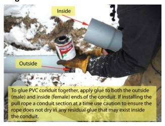
Figure 25—Applying Glue to Conduit
