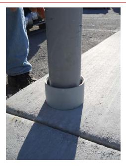
Figure 24—Installing Conduit through Concrete
