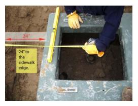
Figure 36-Positioning of a Box Pad
