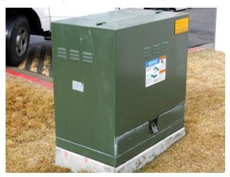
Figure 43—Single-Phase Sectionalizing Cabinet
