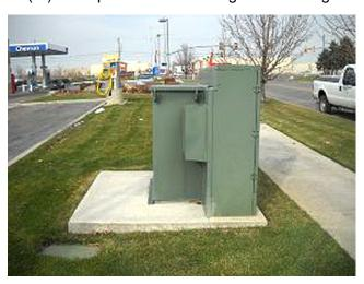
Figure 59—Three-Phase Transformer on a Flat Pad
