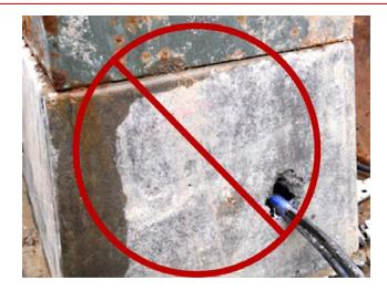
Figure 53—Hole through the Side of a Fiberglass Box Pad
