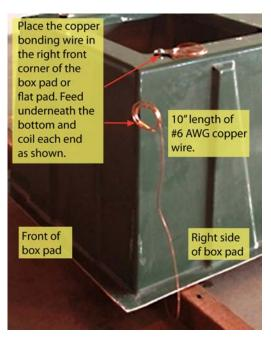
Figure 41-Joint Use Bonding Wire in a Box Pad
