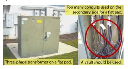
Figure 60—Three-Phase Transformer Flat Pad
