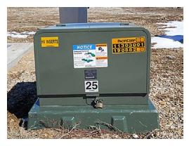
Figure 54—Single-Phase Transformer
