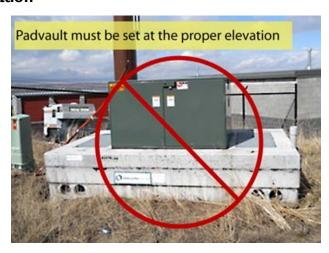
Figure 66—Padvault Not Set at the Proper Elevation
