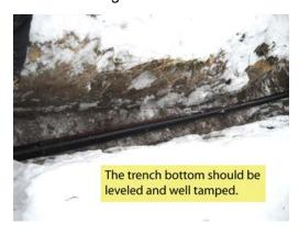
Figure 13—Typical Primary Conductor Trench
