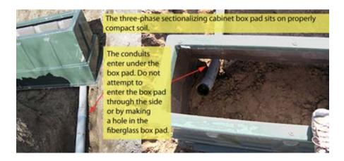
Figure 52—Conduit Placement - Three-Phase Sectionalizing Cabinet
