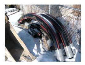
Figure 19—Fiberglass Sweeps
