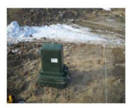
Figure 70—Installed Secondary Box with Pedestal
